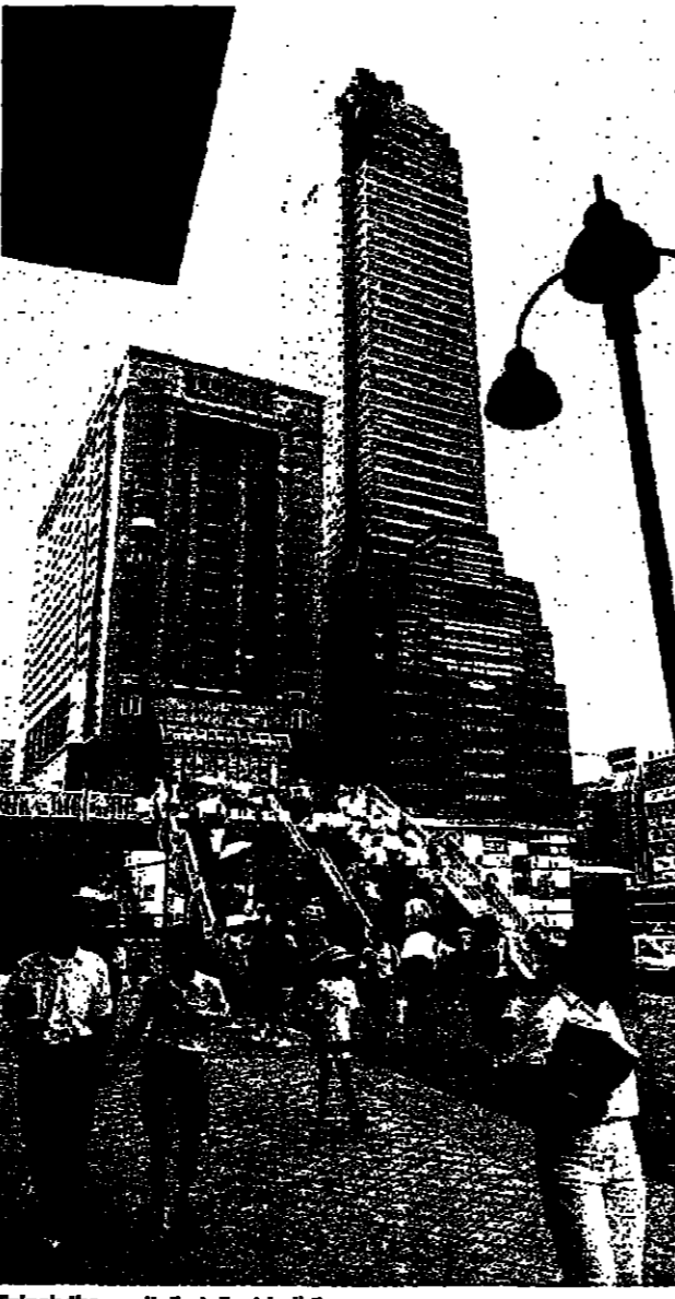
Taipei: the capital's tallest building
